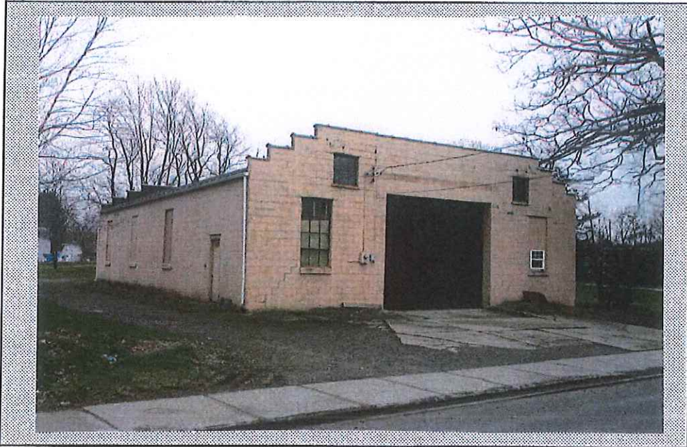
Front view of warehouse
